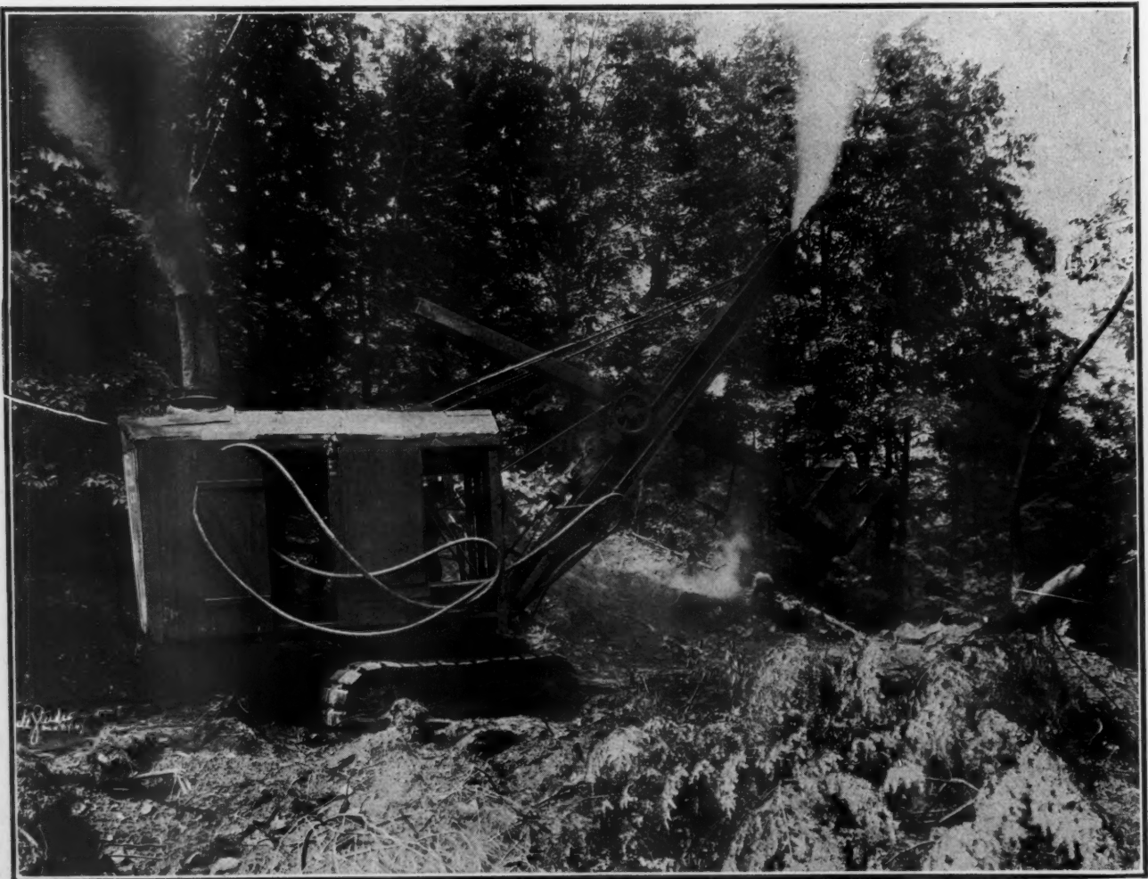
Shovel Stripping and Removing Overburden
